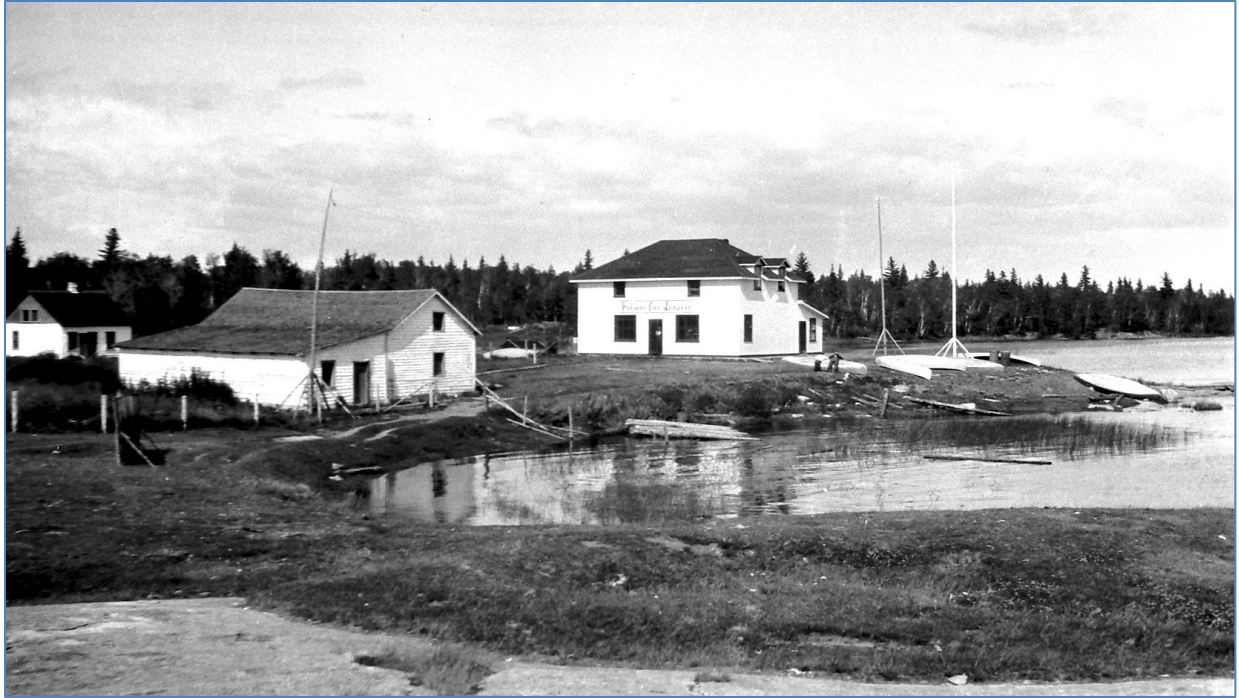
Post buildings at Berens River. (photograph from George Duddy collection)
