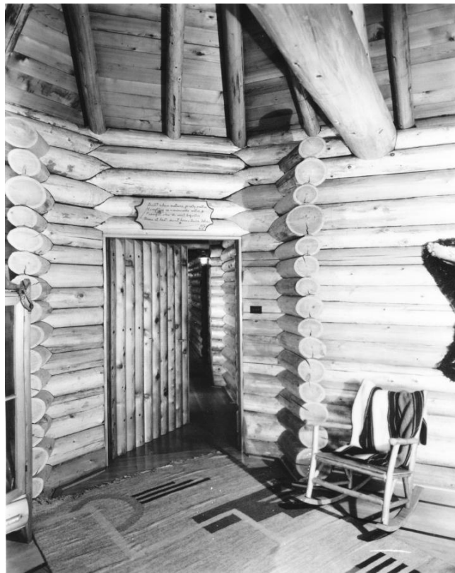
Corner showing log joints with sign above door made by varnishing wool thread onto the wood surface and signed by Alex and Don.
